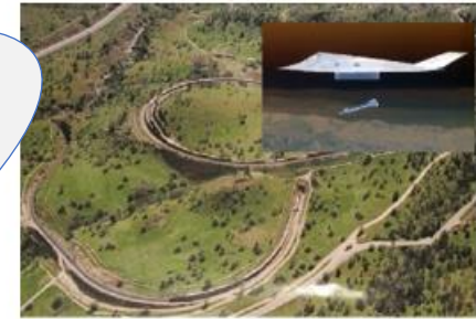
Figure 2. Railway section to be destroyed
